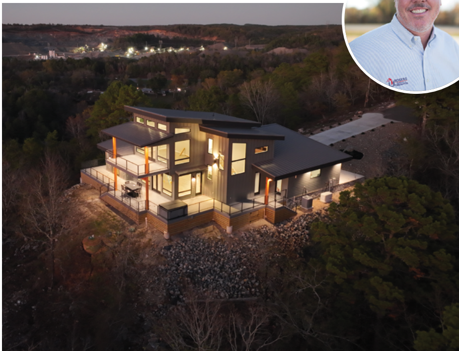
photo courtesy of Rogers Construction
